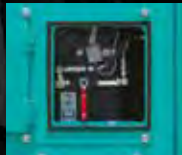
Emergency manual valve for lowering cab
