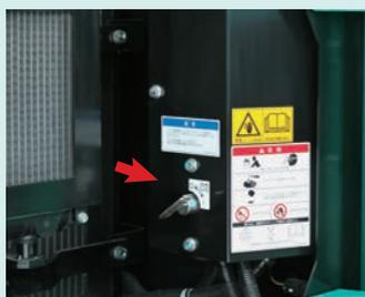
**Battery shut-off device**
